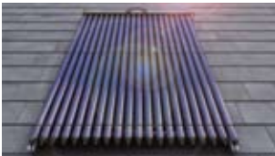
Evacuated Tube Solar Collector
