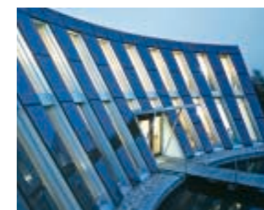
Juwil Offices, Bolanden, Germany
