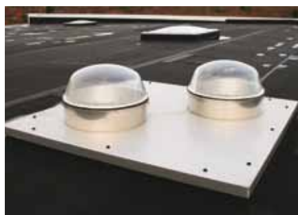
Bespoke flashing for skylight replacement (not a Solatube product)
